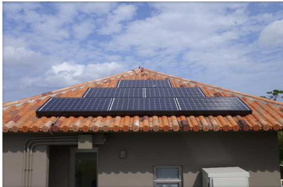
(a) PV panels equipped on the roof of each house.
